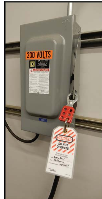
Figure 1: Lockout/Tagout on the Power Source Panel
