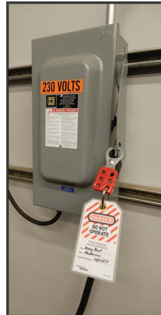
Figure 1: Lockout/Tagout on the Power Source Panel
