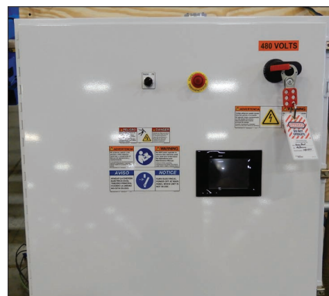
Figure 2: Sample of a Lockout/Tagout Mechanism on an Electrical Enclosure
