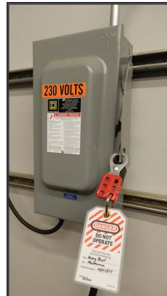
Figure 1: Lockout/Tagout on the Power Source Panel
