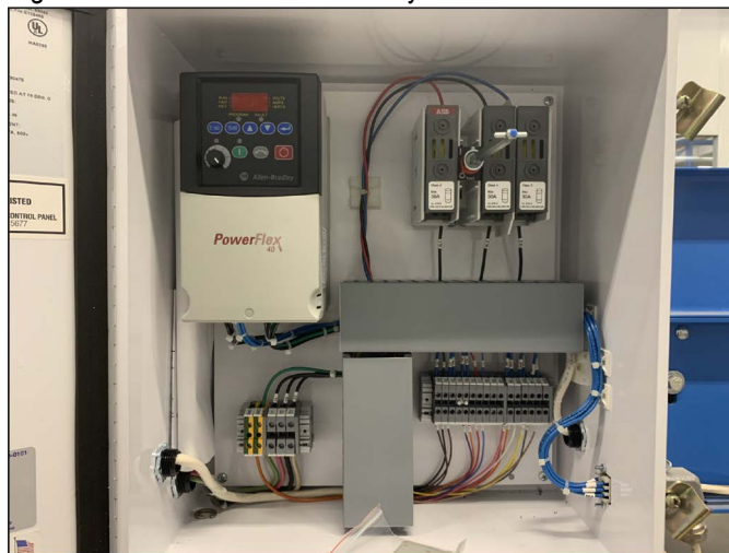
Figure 2: Powered Skewed Conveyor Enclosure
