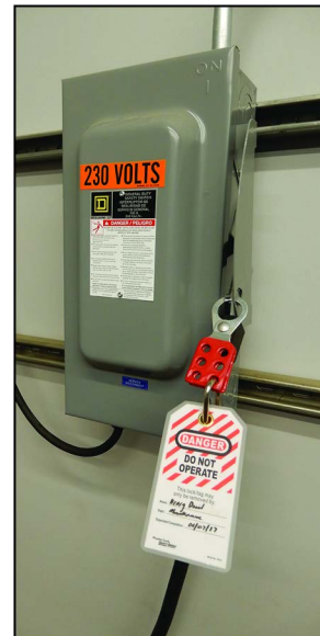
Figure 1: Lockout/Tagout on the Power Source Panel
