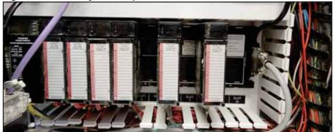
Figure 20: Carriage-End Output Modules Removed
