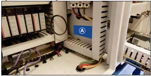
3. Drill and tap holes for the DIN rail. The holes should be 3-1/2" above the bottom wire duct.
