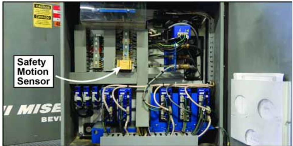
Figure 3: Safety Motion Sensor in Secondary Electrical Enclosure
