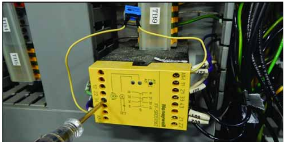
Figure 4: Removing Wires
