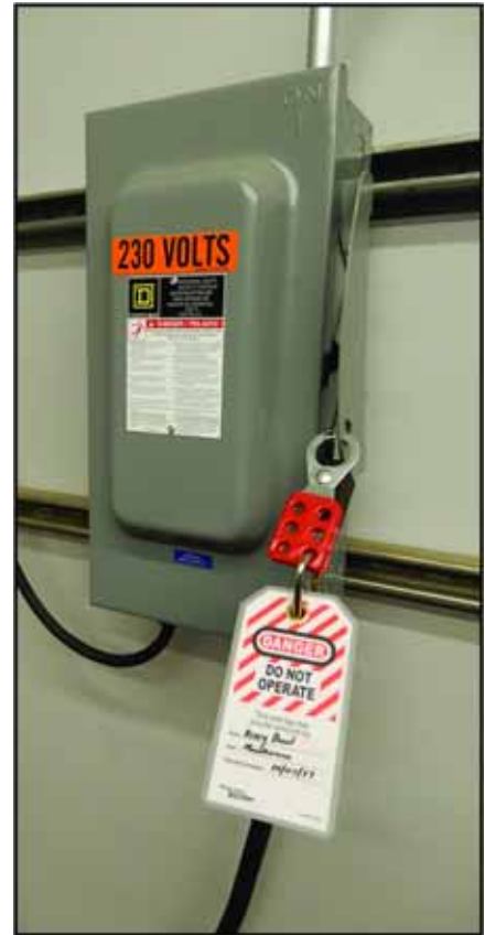
Figure 2: Lockout/Tagout on the Electrical Service Entry Panel
