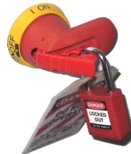
Figure 1: Lockout/Tagout on the Main Electrical Enclosure
