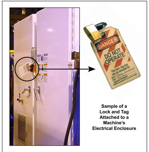
Figure 4-1: Lockout/Tagout on the Main Electrical Enclosure
