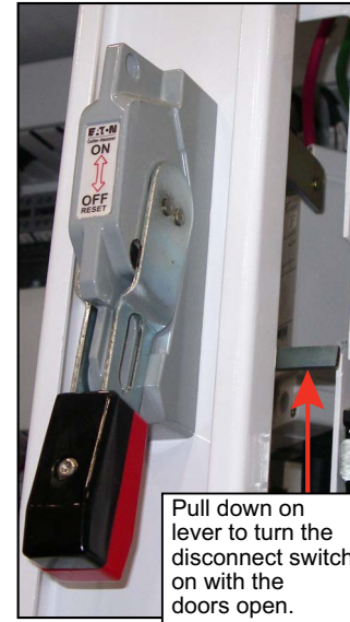
Figure 2-69: Turning On the Disconnect Switch
