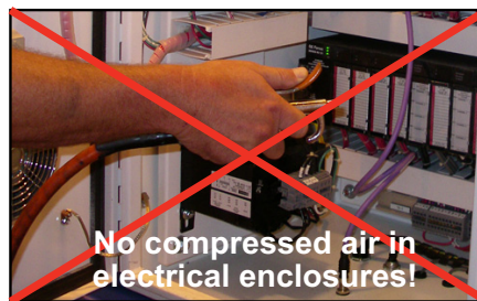
Figure 2-19: Never Use Compressed Air Inside an Electrical Enclosure
