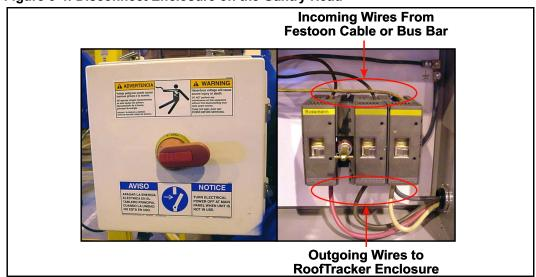
Figure 3-4: Disconnect Enclosure on the Gantry Head
