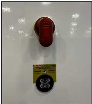
Auto Deck Disconnect Switch
