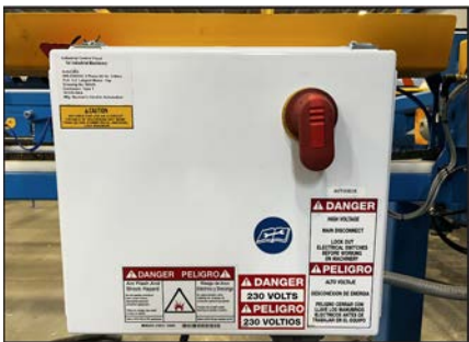
Auto Deck Disconnect Switch
