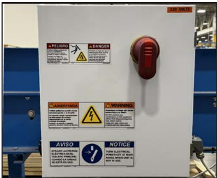
Skewed Conveyor Disconnect Switch
