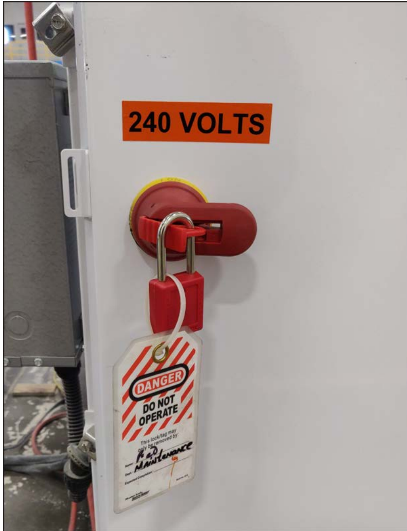
Figure 1-2: Example of a Lockout/Tagout Mechanism on an Electrical Enclosure
