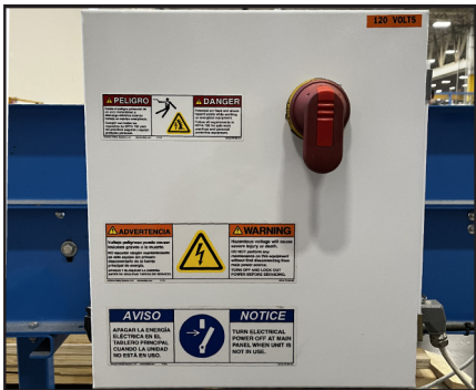
Skewed Conveyor Disconnect Switch
