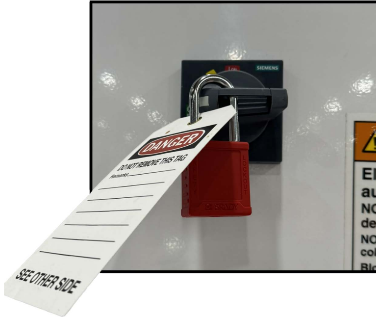
Figure 1-2: Example of a Lockout/Tagout Mechanism on an Electrical Enclosure
