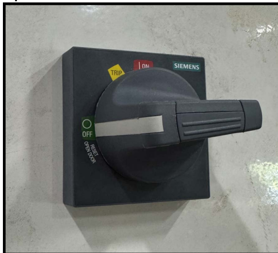
Figure 1-1: Example of a Disconnect Switch in Off Position
