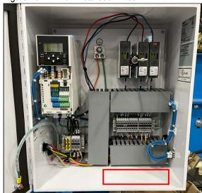
11. Before connecting wires to the Timer, make sure that all DIP switches are configured in the down position as shown in Figure 11.
