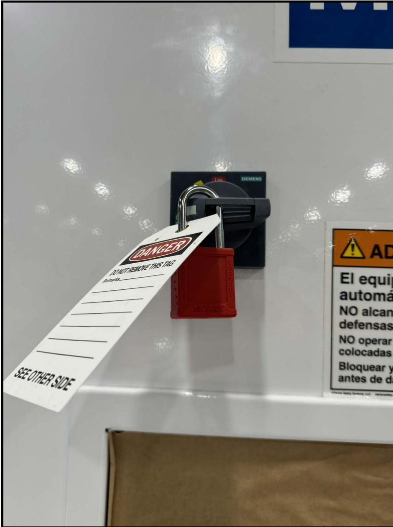
Figure 1-2: Example of a Lockout/Tagout Mechanism on an Electrical Enclosure
