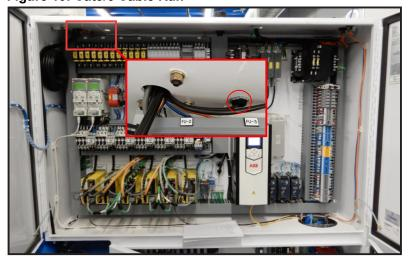
d) In order to ease the process of fishing the **50-ft Cat5/6 cable** (i.e. connecting two cables together to pull one through an existing cable run), remove the connector end of the **USB cable for Moxa converter.** Then connect the bare end of the **USB cable for Moxa converter** to the **50-ft Cat5/6 cable** with electrical tape.
