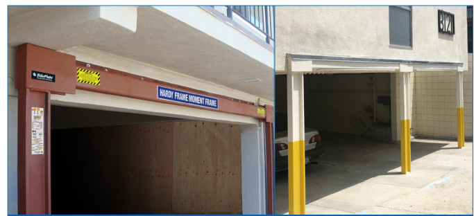
SPECIAL MOMENT FRAME IN RETROFIT APPLICATIONS
