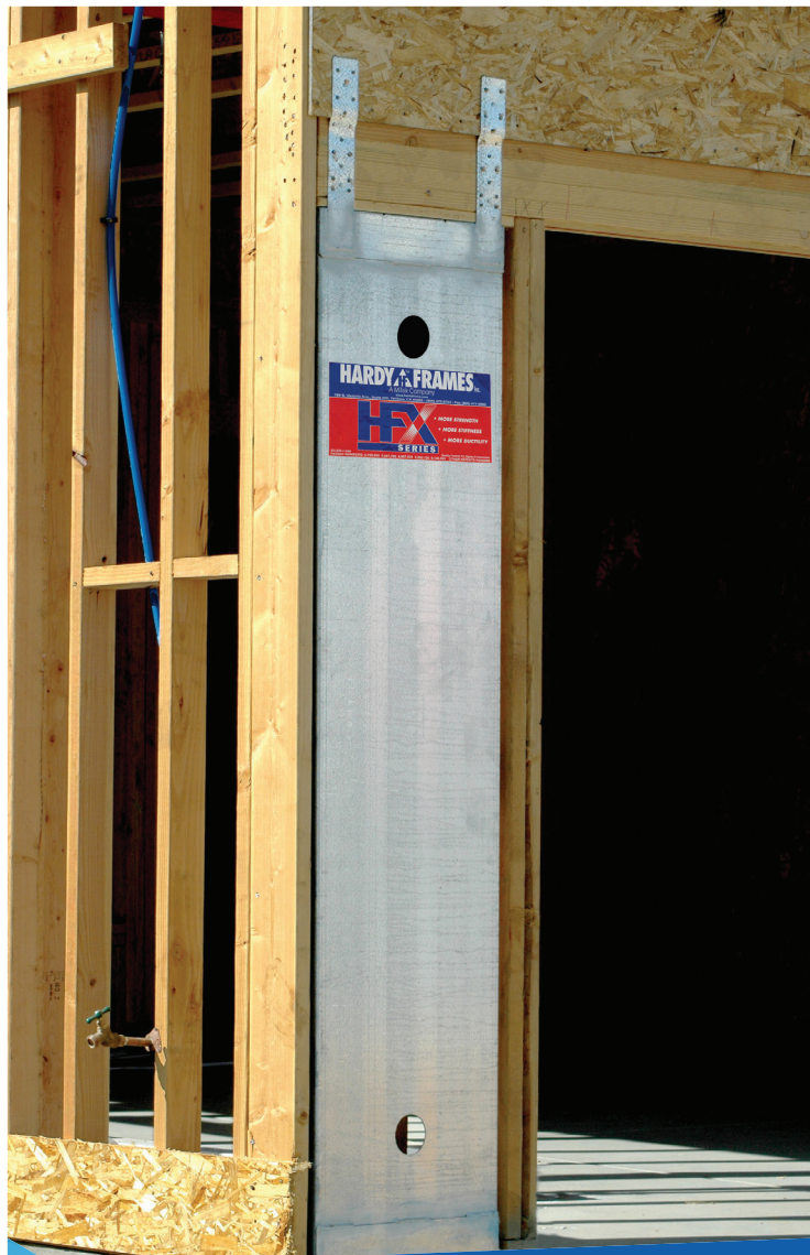
GARAGE FRONT WITH STRAPS
