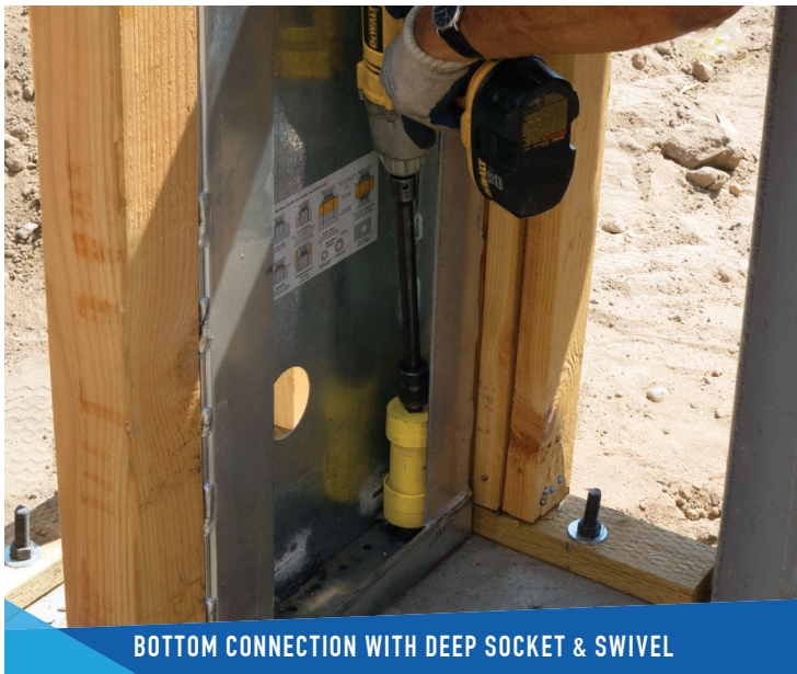
PORTAL INSTALLATION WITH SOFFIT & FIXTURES
