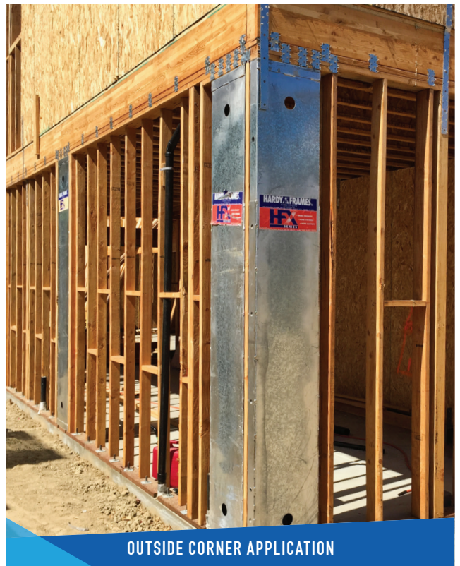
GARAGE FRONT WITH STRAPS
