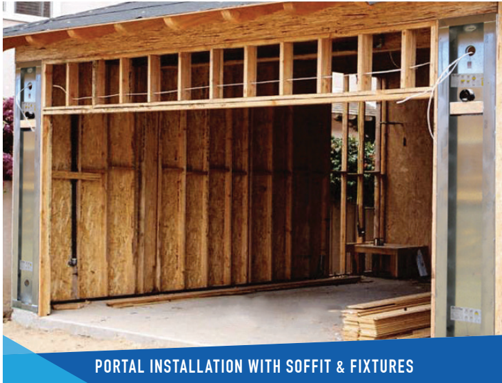
GARAGE FRONT HANGING SOFFIT
