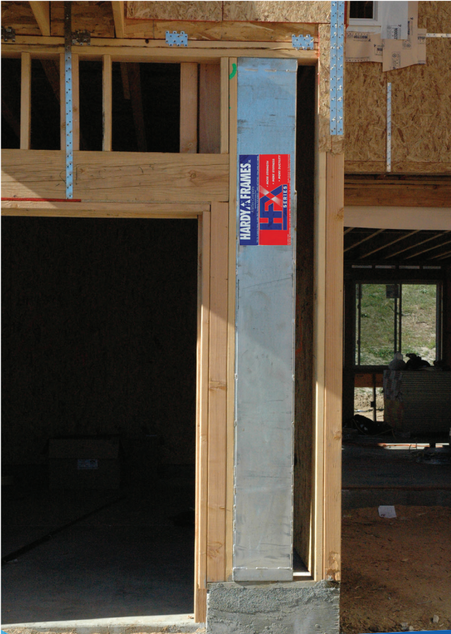
GARAGE FRONT TOP PLATE CONNECTION
