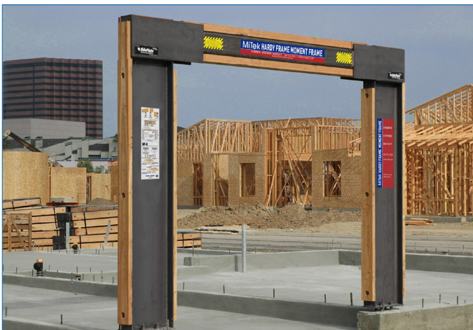
SPECIAL MOMENT FRAMES NEW CONSTRUCTION
