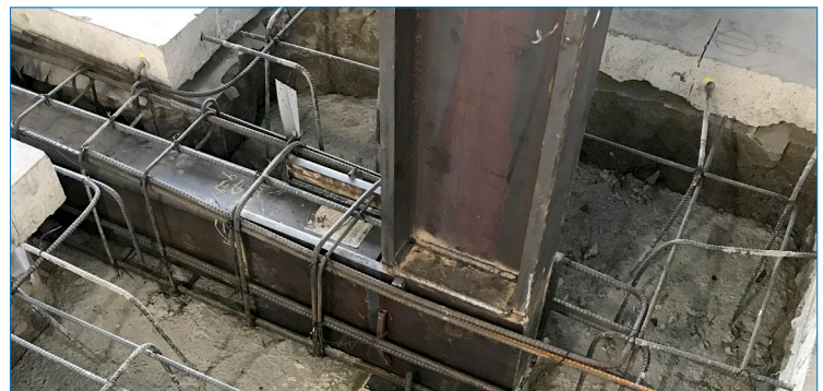
PICTURE FRAME WITH FOUNDATION BEAM INSTALLATION
