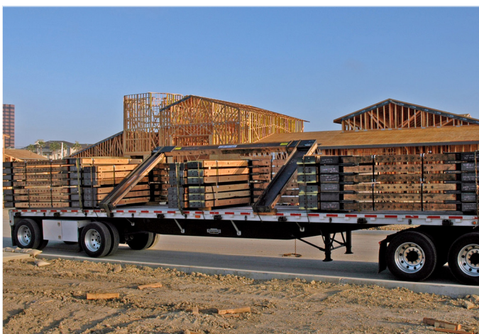
SPECIAL MOMENT FRAMES DELIVERY TO JOB SITE
