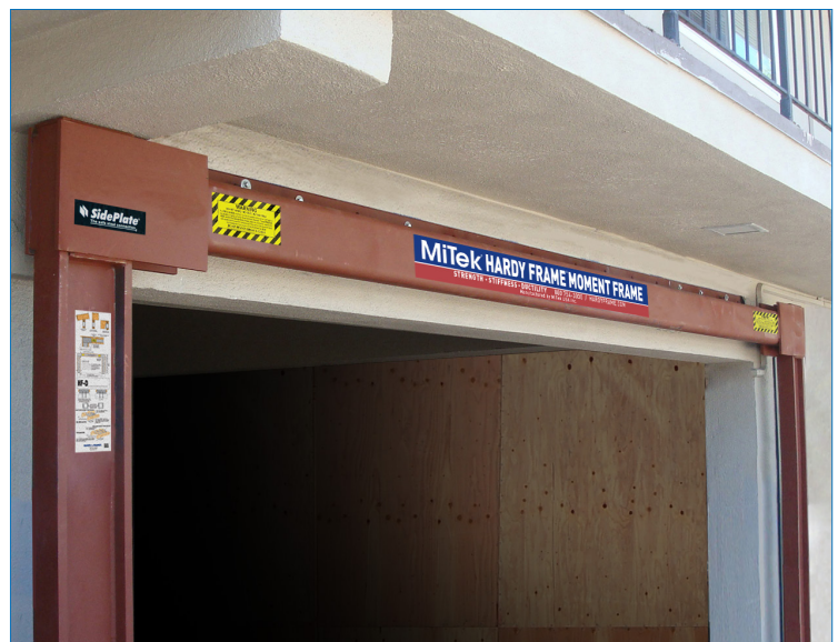
SPECIAL MOMENT FRAME IN RETROFIT APPLICATIONS
