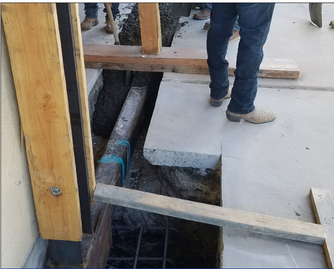
INSTALLING HARDY FRAME PICTURE FRAME
