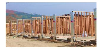
Two MiTek brands (Hardy Frame® Shear Wall System and USP Structural Connectors) were chosen for use in the 1,200-apartment, 47-unit luxury apartment development in southern California. A total of 465 shear walls were installed, along with \$250,000+ worth of USP hangers, connectors, and straps.
