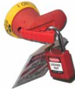
Figure 1: Lockout/Tagout on the Main Electrical Enclosure
