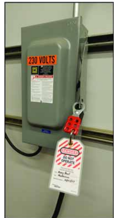
Figure 1: Lockout/Tagout on the Power Source Panel
