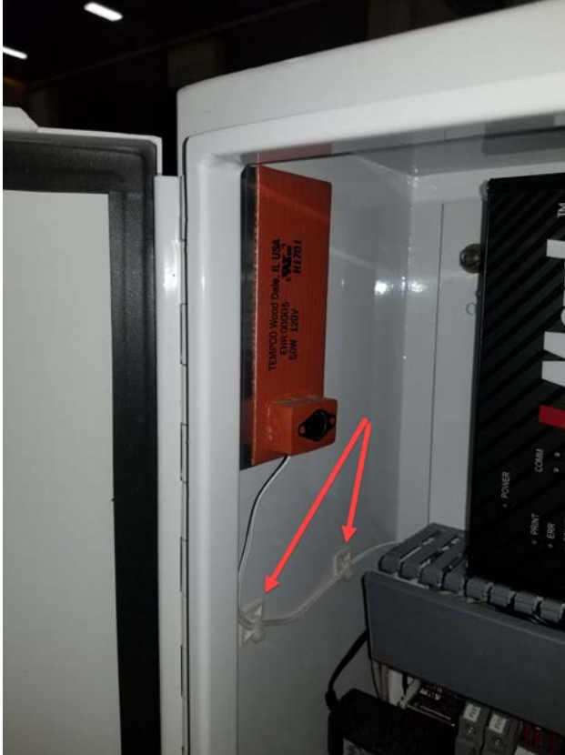
Figure 6: MPA Tie Wrap Pad Approximate Placing
