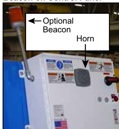
Figure 8: Horn and Optional Beacon on Control Panel
