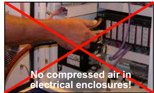
Figure 7-2: Never Use Compressed Air Inside an Electrical Enclosure
