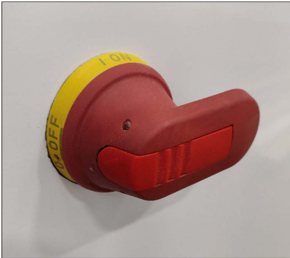
Figure 1: Disconnect Switch in Off Position
