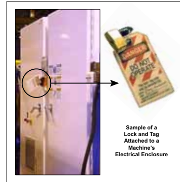
Figure 1: De-Energizing Electrical Power at the Machine's Disconnect Switch
