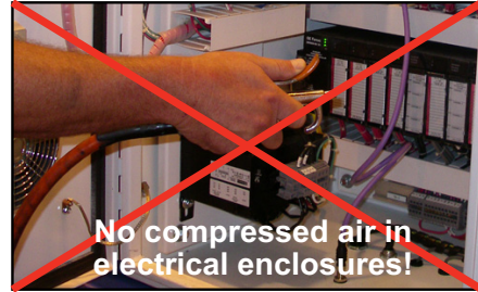
Figure 6-5: Never Use Compressed Air Inside an Electrical Enclosure
