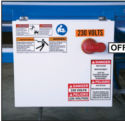
Figure SAFETY-2: Lockout/Tagout on Additional Equipment in the System
