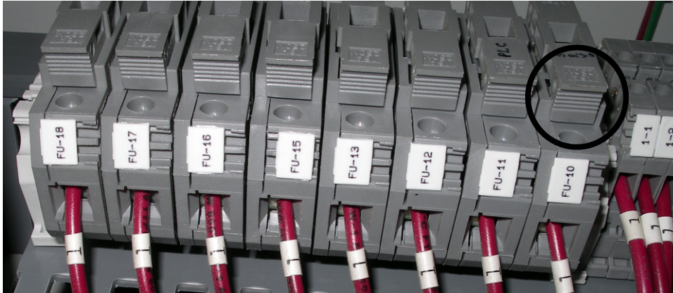
Figure 2-88: Fuse on Top of Terminal Block (view from side)
