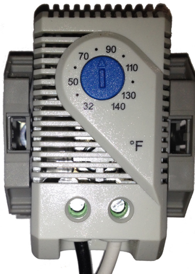
Figure 2-58: Thermostat Inside the Touch Screen Enclosure
