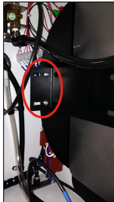
Figure 2-99: Remove the Touch Screen Bracket Screws
