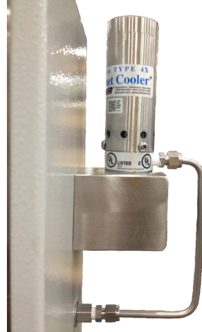
Figure 2-57: Cooler on Outside of Touch Screen Enclosure
