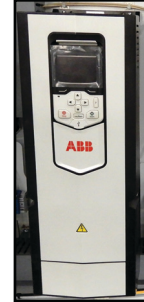
Figure 2-81: Primary VFD
