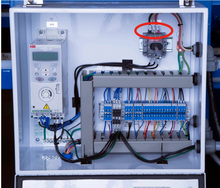
Figure 2-17: Swap 2 of the 3-Phase Wires to Change Motor Direction on Auto Deck
