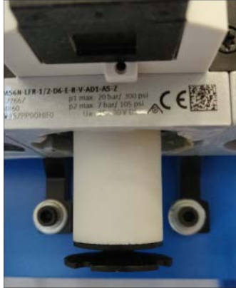
Figure 7-64: Filter Element with Bowl Removed
