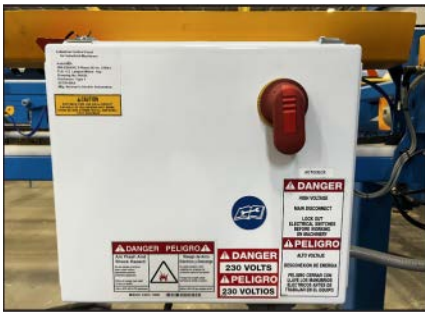
Auto Deck Disconnect Switch
