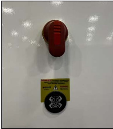
Auto Deck Disconnect Switch
