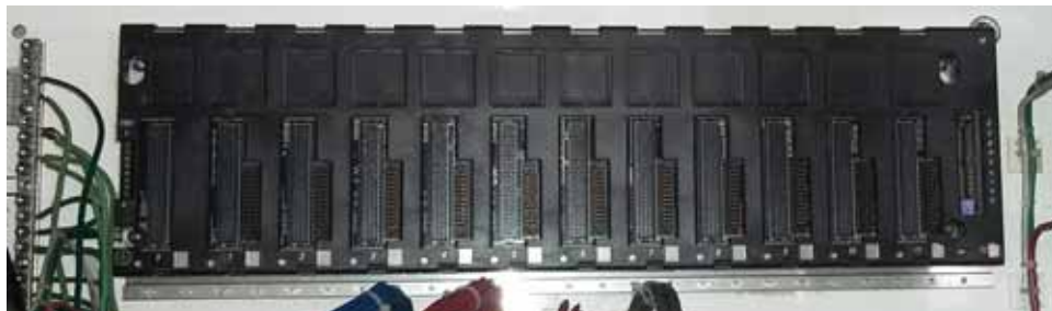
Figure 11: New Backplane Installed
