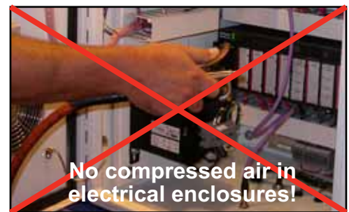
Figure 7-16: Never Use Compressed Air Inside an Electrical Enclosure
