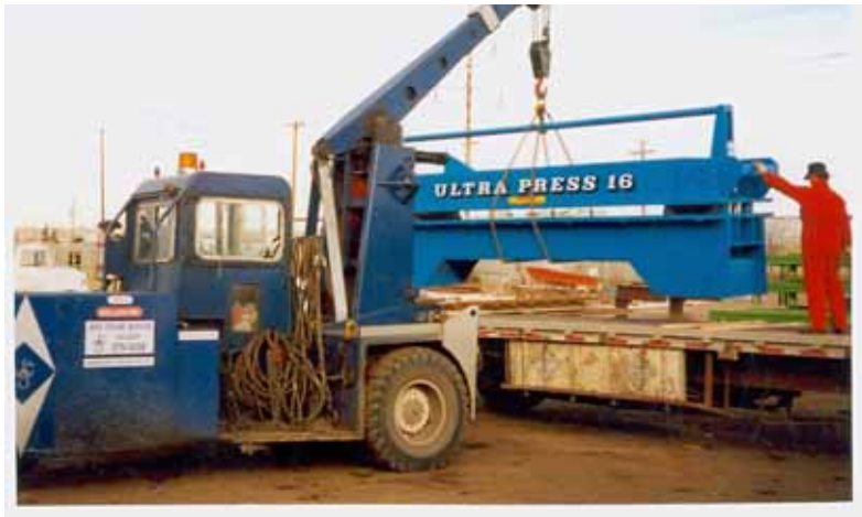
Unloading Ultra-Press With Mobile Crane (25 Ton Capacity)
