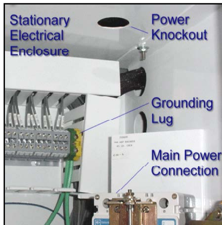
Figure 3-17: Disconnect Enclosure
