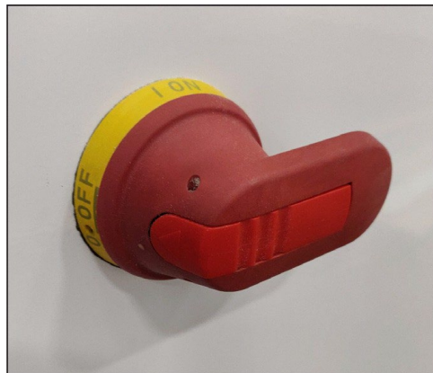
Figure 1-1: Disconnect Switch in Off Position
